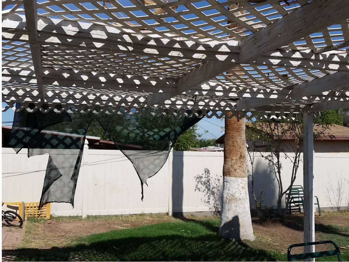
Patio Cover Renovation Potential Enhancement to Project If Budget Permits
