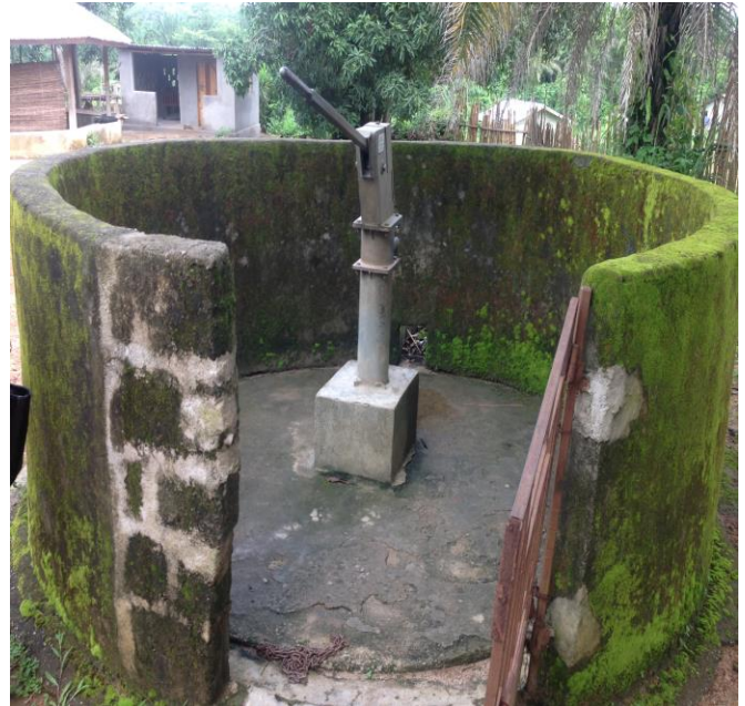
Inoperable mechanical water well located next to the health clinic. This water well was bypassed. It works intermittently. All indicators points to this well simply not dug deep enough. We will fix this problem next year after rainy season providing we have the resources to complete do the job.
