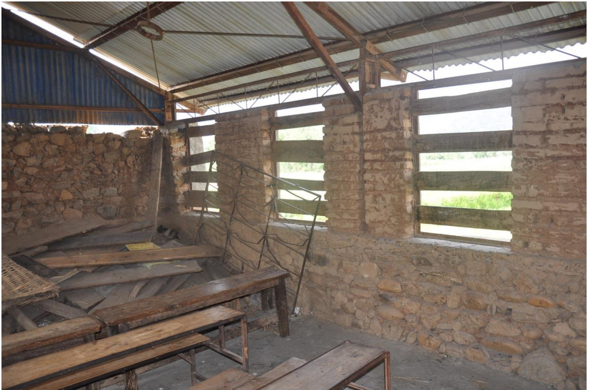
Another view of room to be renovated in Sindhuli district school.
