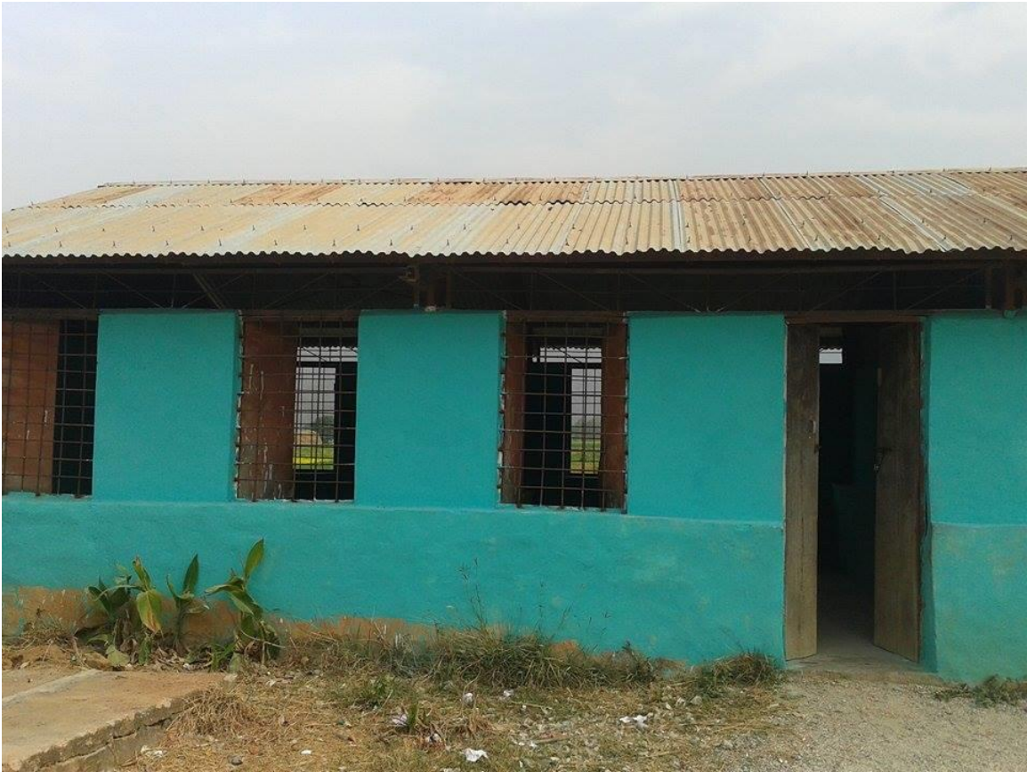
Classroom after reconstruction.
