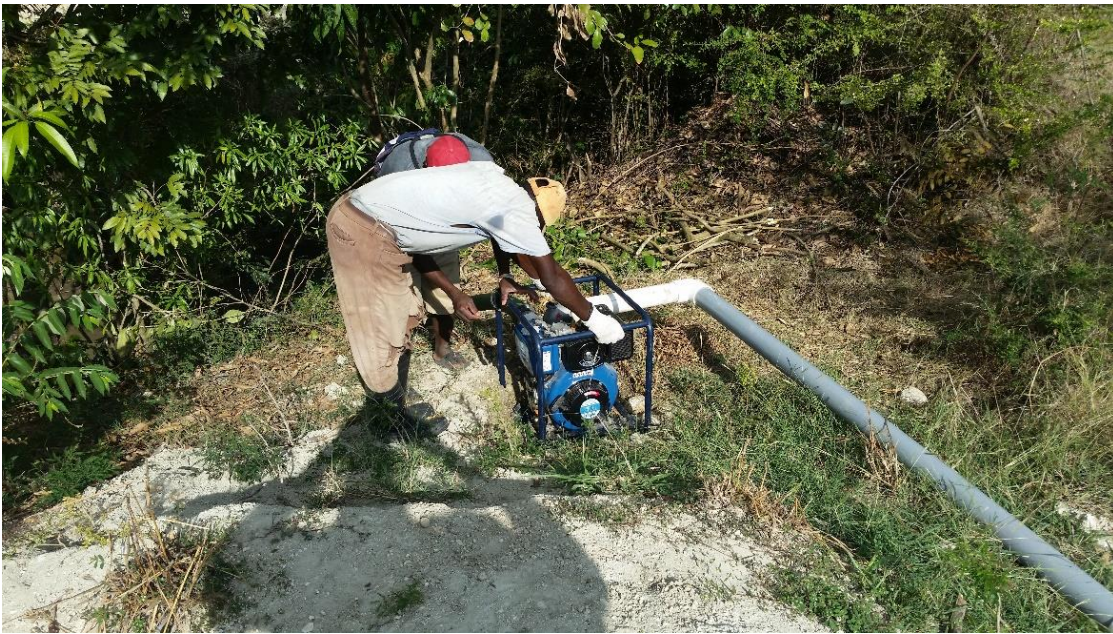
Rotary purchased pump being installed and put into place.
