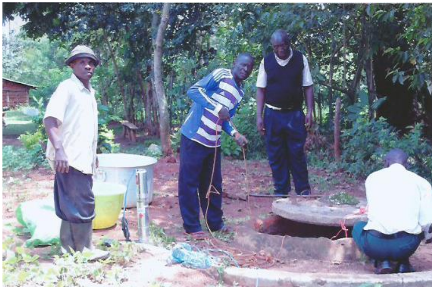
REPAIRING OF BROKEN BOREHOLE.
