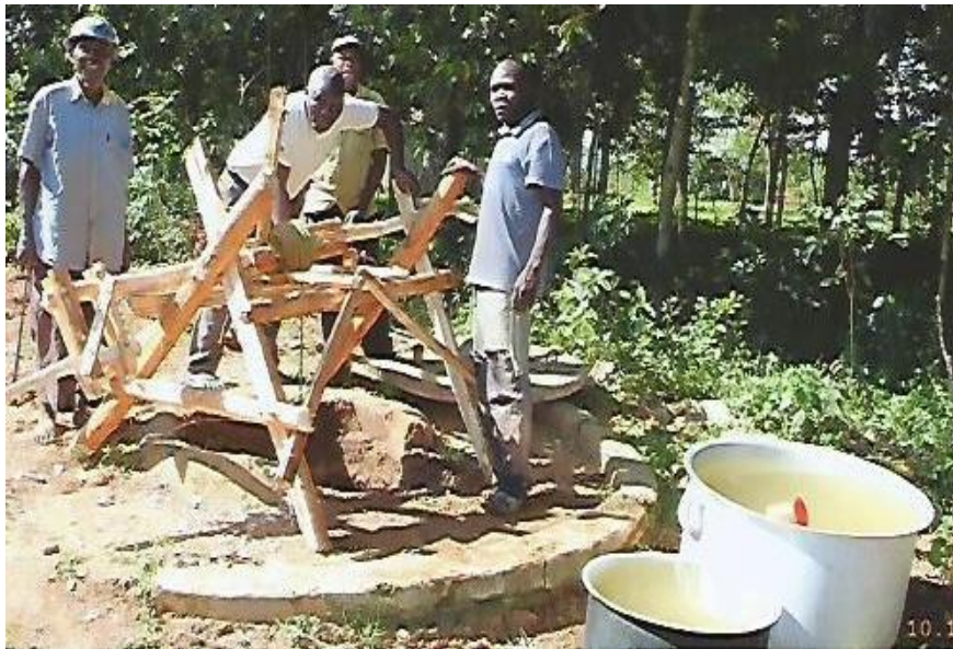
REPAIRING OF BROKEN BOREHOLE
