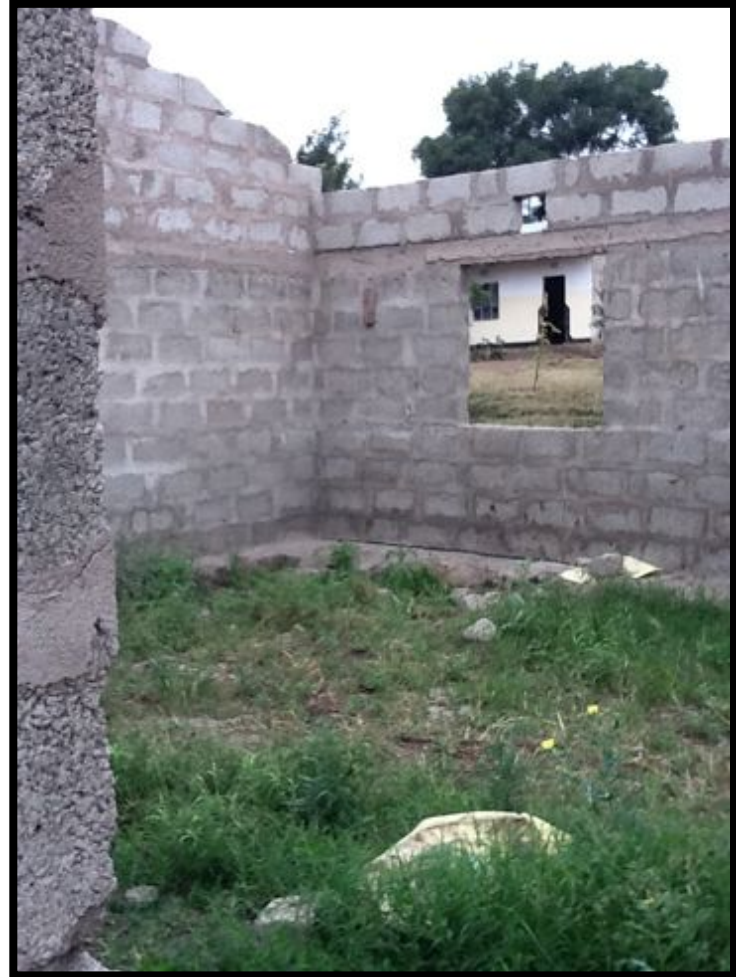
The Current Interior of the Classrooms (no floor)
