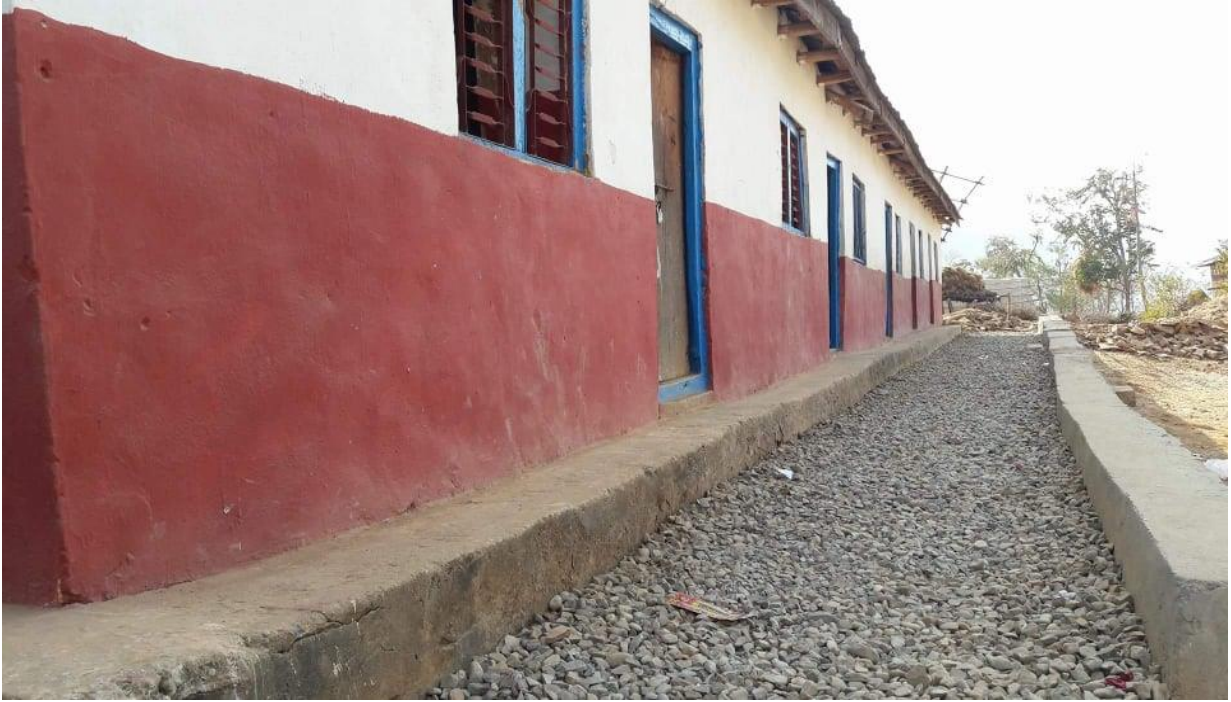
School Building. Five rooms were reconstructed
