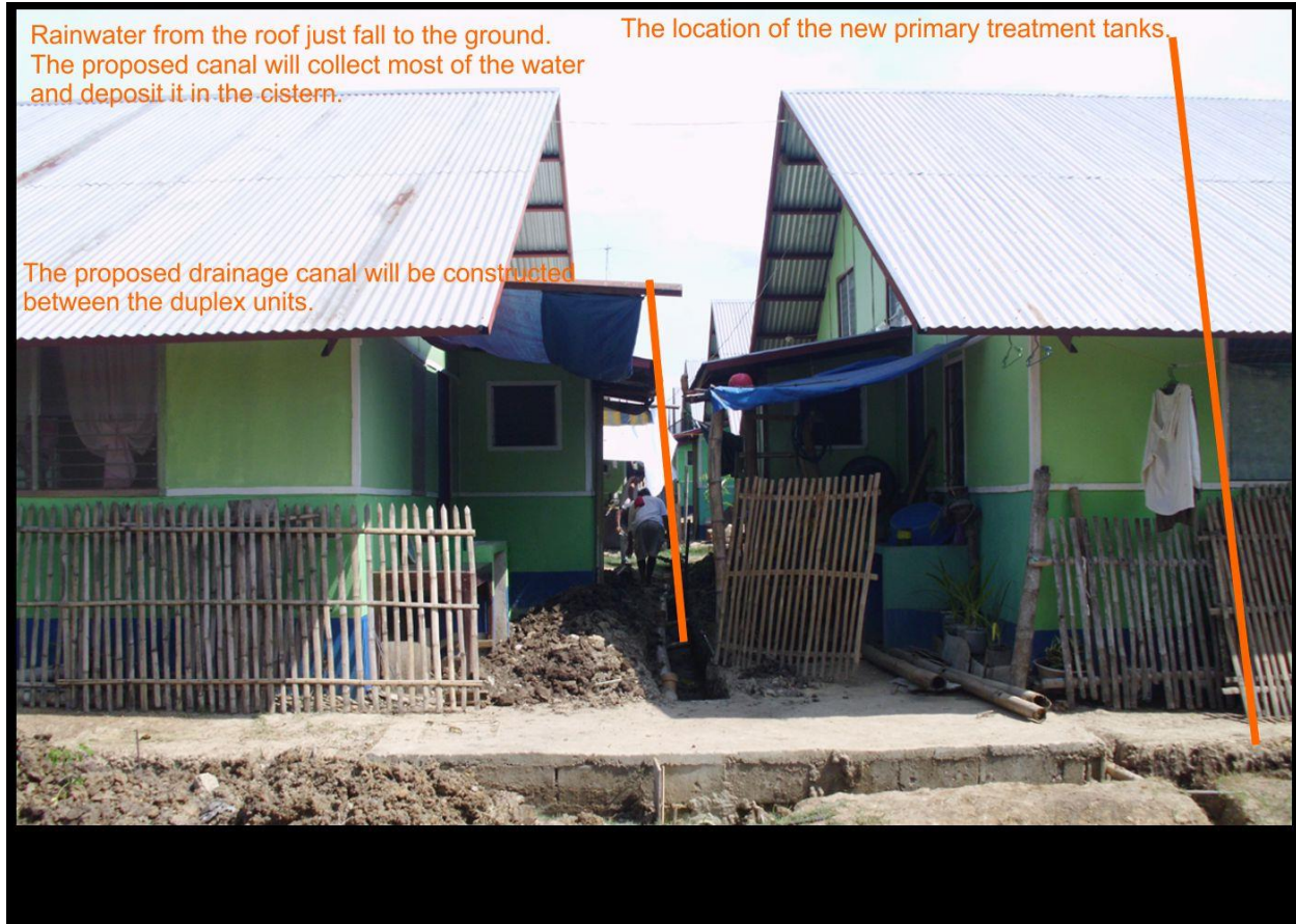
Picture No. 5: Rainwater harvesting potential of drainage canal in combination with greywater line.
