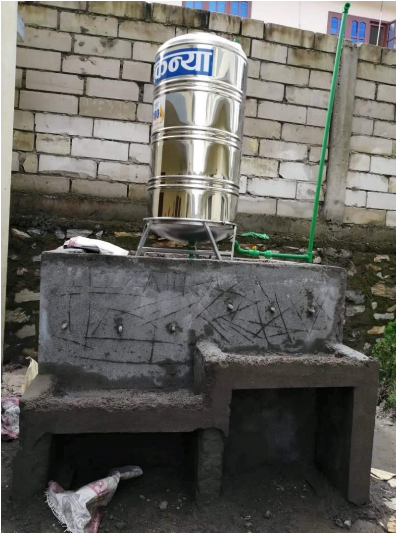
Constructing new distribution facility with new piping, filtration, and storage tank.
