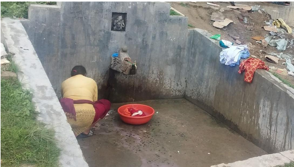
Water supply before reconstruction of supply piping and terminal filtration facilities.
