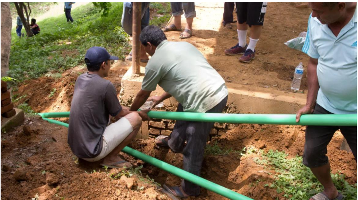
Laying new pipe to water distribution terminal
