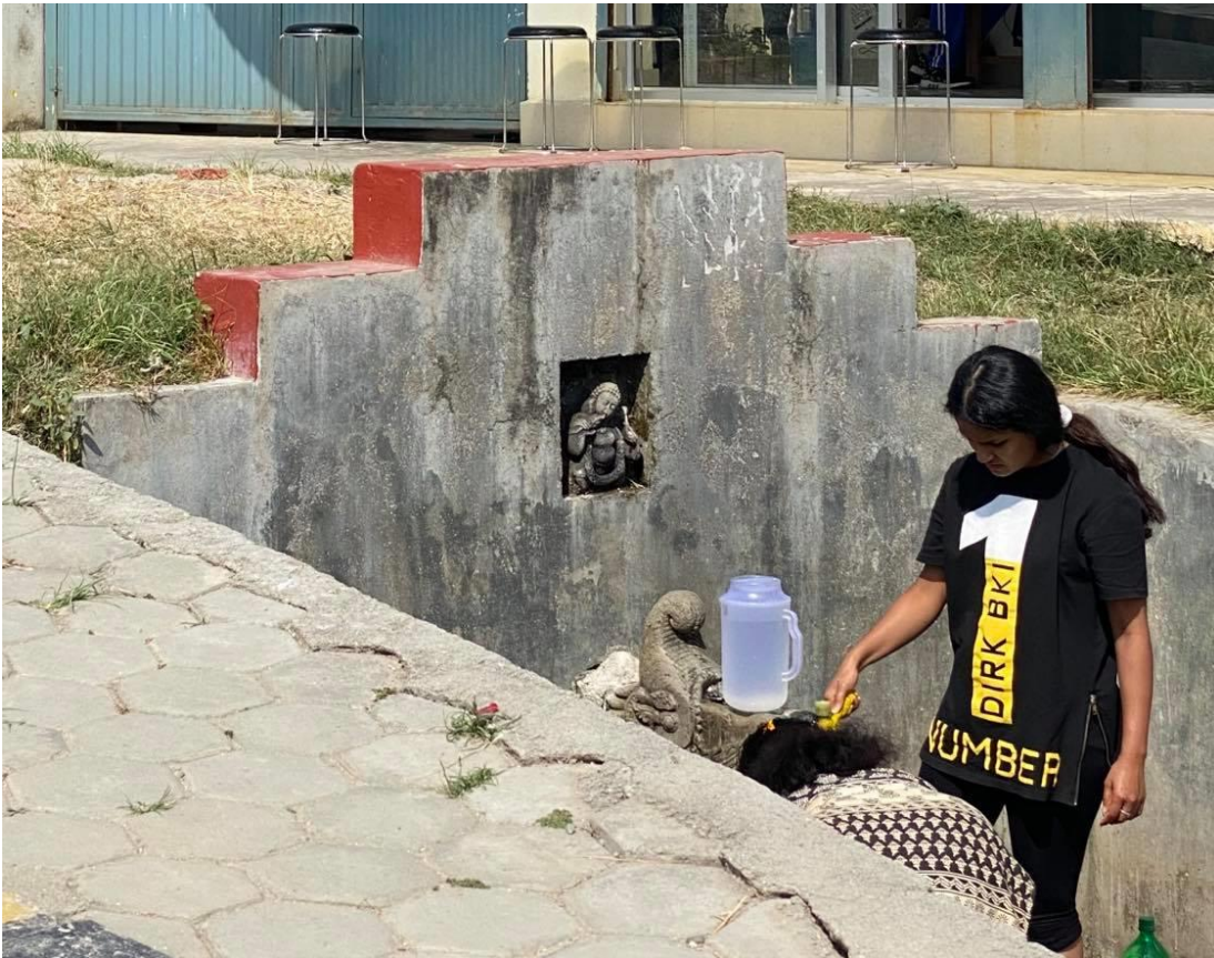
Original water supply facility.
