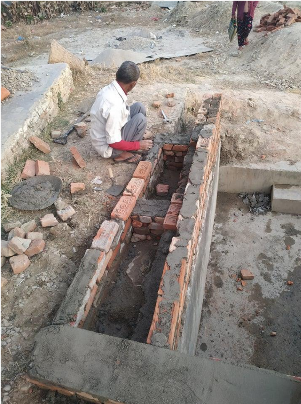
Rebuilding water supply facility
