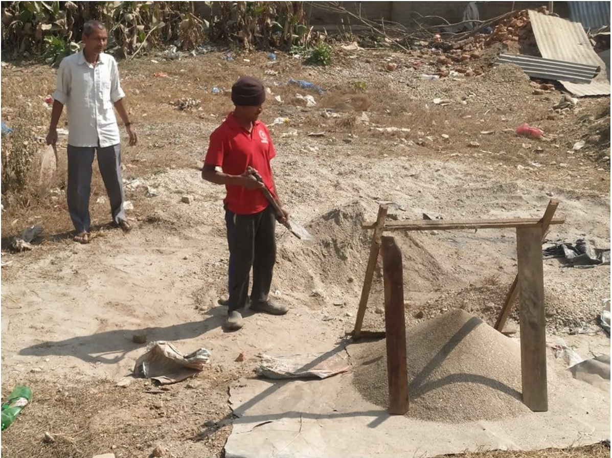
Sand used for reconstruction.
