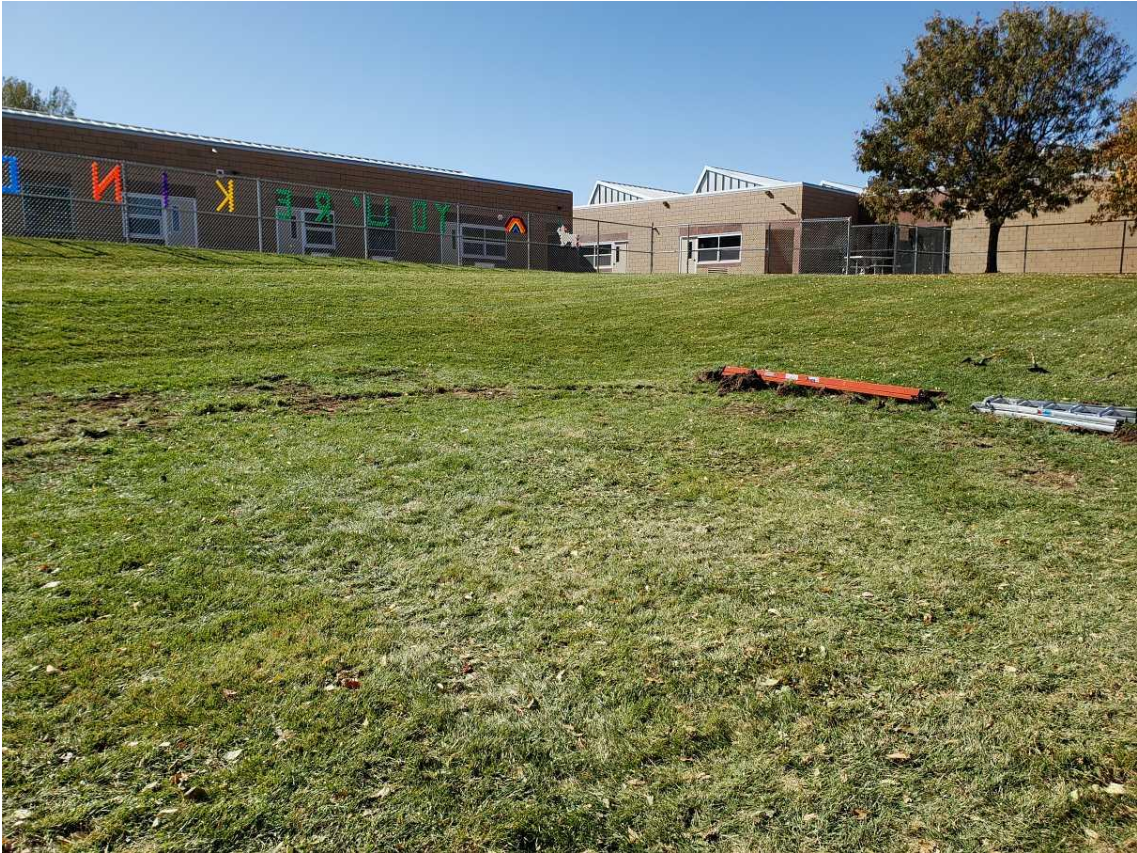
Mission accomplished. Backstop removed.
