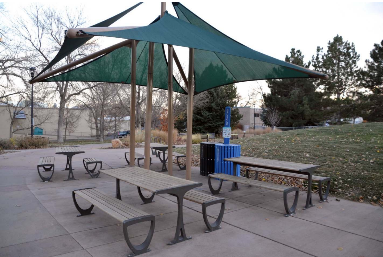
Picnic tables under new shelter.
