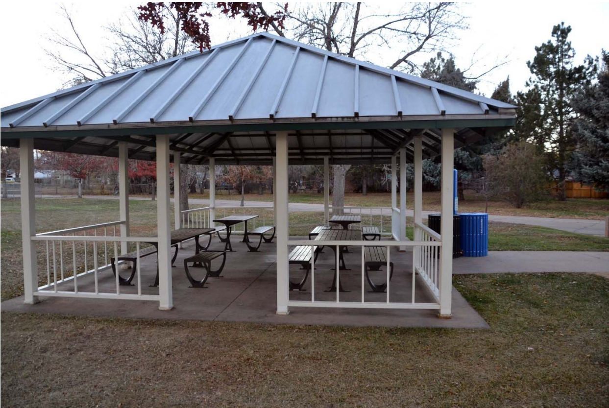
Pre-existing shelter with new picnic tables.
