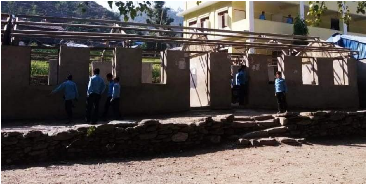
Shree Bac School with new structural steel in roof.
