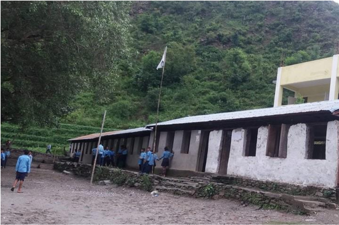
Shree Bak School before repairs.
