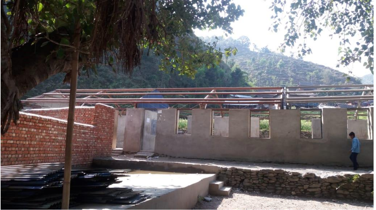
Shree Bac School during repairs.
