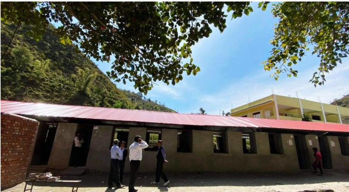
Shree Bac School with repairs nearly completed.
