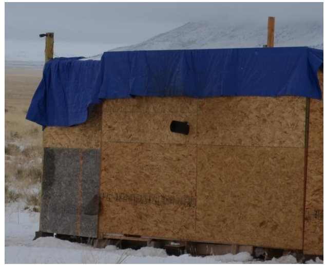
Note the tarp use for a roof ^ and the stove pipe.
