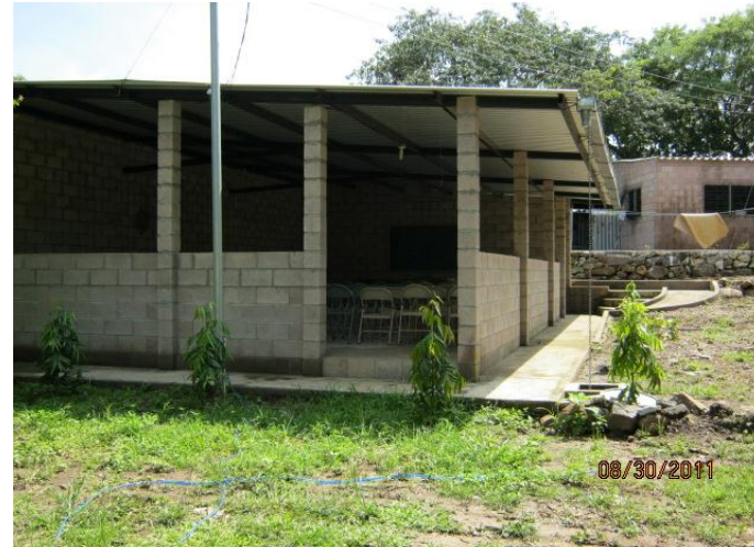
Auditorium for trainings
