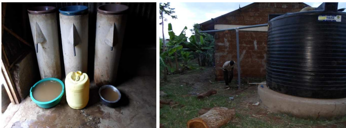
Some of the filters that were installed yet to mature at GachuaPri and a complete RWH system.
