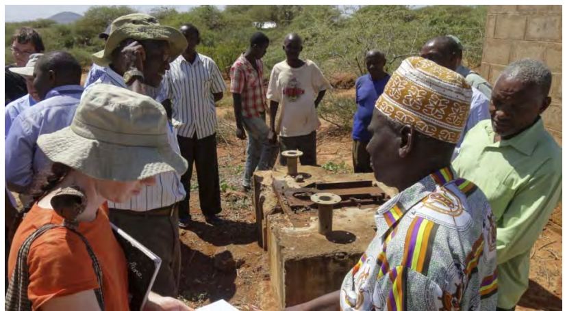
Learning from a borehole that failed after 2 years
