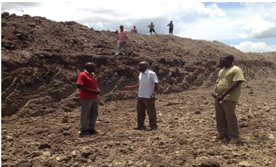
Site visit on 05/April/2014 between Eng Batumbya and WGUL field staff.
