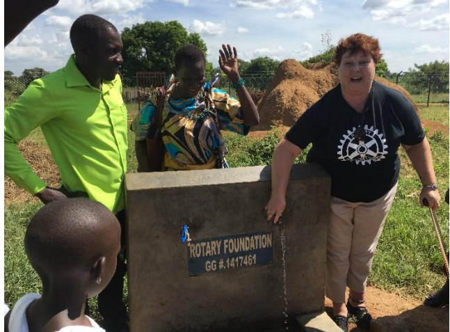
Solar powered water - Ugandan GG project 2016
