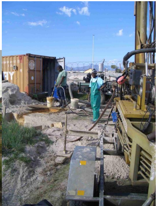
Borehole being installed on the SCAGA site.
