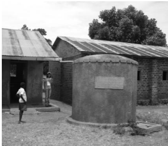
Figure 3.12 Rainwater Catchment - Ferrocement
