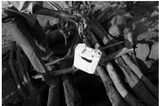
Figure 3.3 Unlined Well
