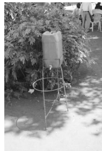
Figure 4.5 Hand Washing Station
