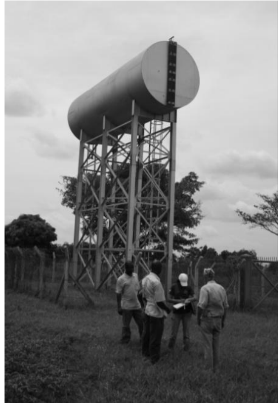
Figure 3.8 Nankoma Village Water Tank
