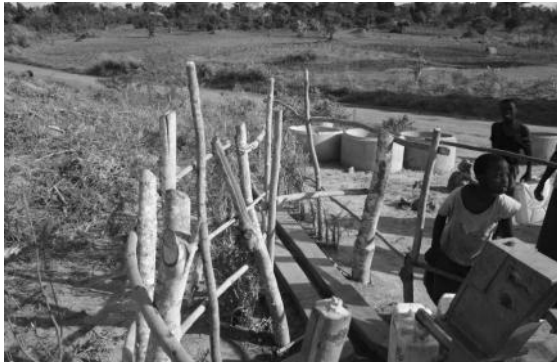
Figure 3.4 Lined Well With Handpump
