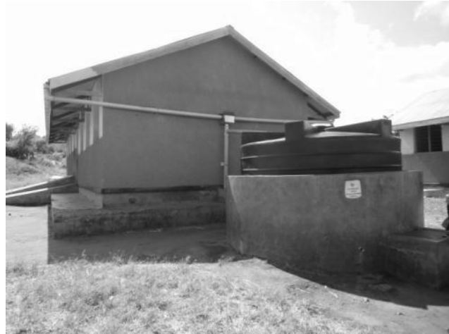
Figure 3.11 Rainwater Catchment - Plastic
