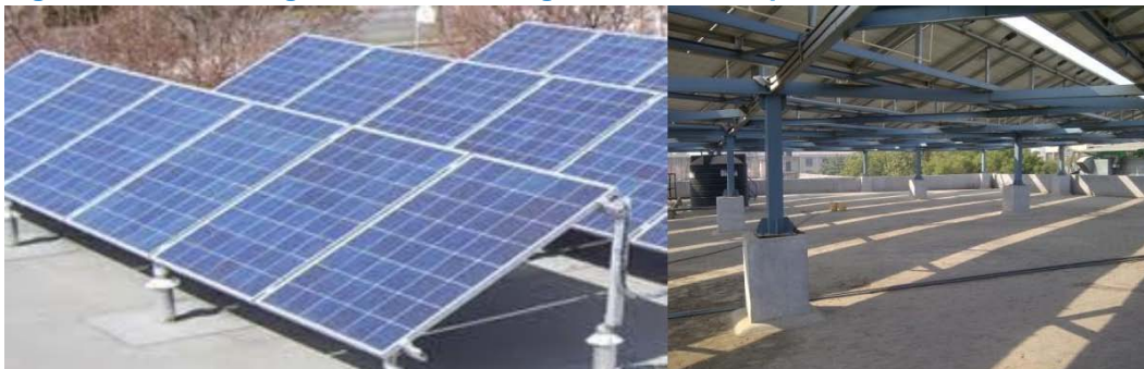
Figure 3 – Lower height and Raised height installation options:
