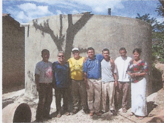
A start – one of two tanks constructed in August/September
