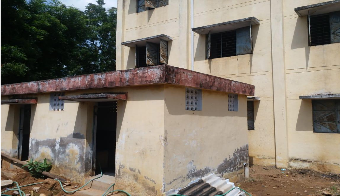
Pic 3: View of toilet Block available at present within campus
